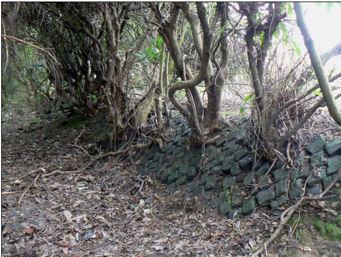
Plate 18: Stone revetment forming the northern side of the sunken feature
